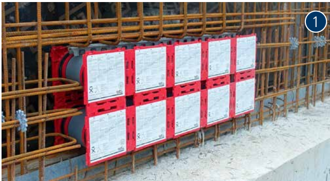
double wall insert HSI150 K2 before concreting
