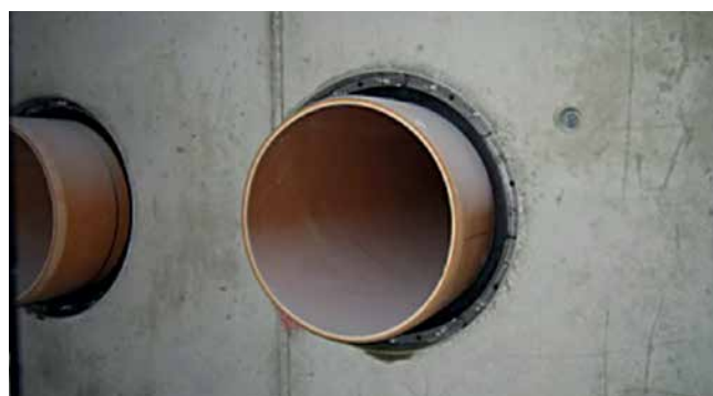
HSD500 G 1x429 b40 A2/EPDM55 Aération/ventilation
