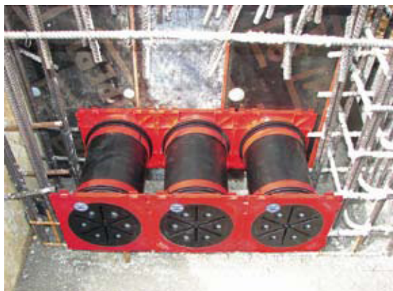
Fig. 4 Tongue- and groove technique at the flange edges for simple formation of a kit assembly of HSI 150 lead-throughs.
