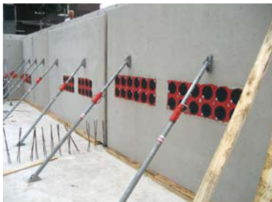
Fig. 7 Use of HSI 150 cable lead-throughs in precast walls.
