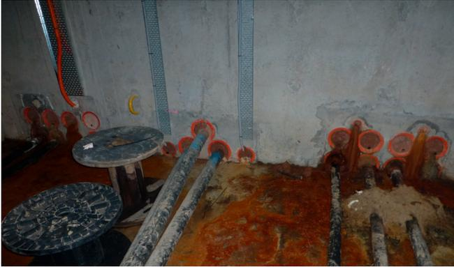
Passive fire protection materials washed out of the penetrations and water damaged the steel footings
