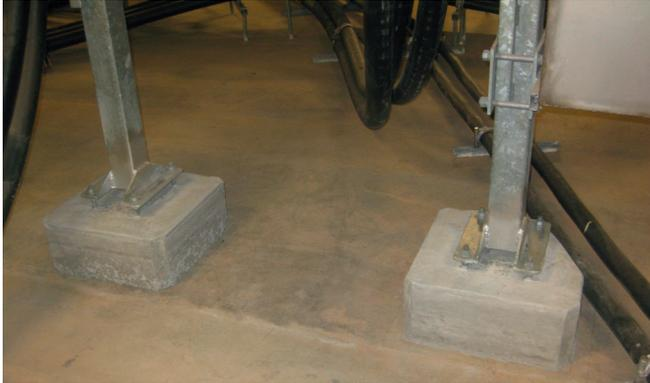
Concrete footings installed to raise steel works off water level
