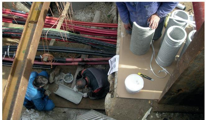
Installation of the split fibre cement sleeves FZR-G.
