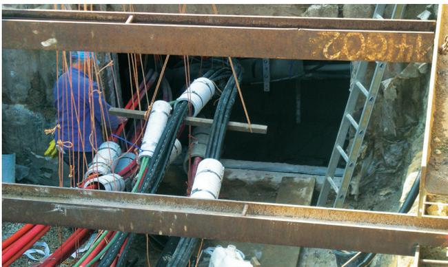
An opening was created around the existing cables and wall sleeves and a split wall sleeve was installed around each cable system.
