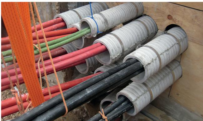
The cable systems were fixed with ropes to secure them in the correct position within the framework.
