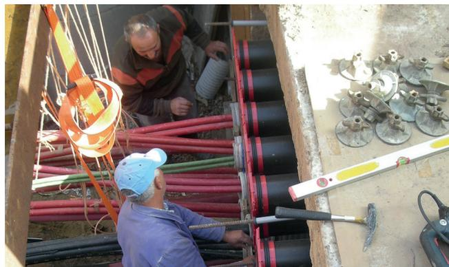
Installation of wall inserts HSI 150-K2 and the split wall sleeves FZR-G.
