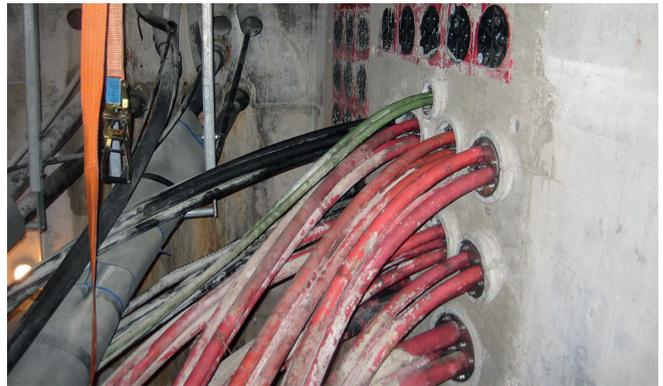
Siphon water intake after redevelopment: spare openings were created. Split wall sleeves were installed around the cables already laid which ensured the tightness between wall, wall sleeves and cables.
