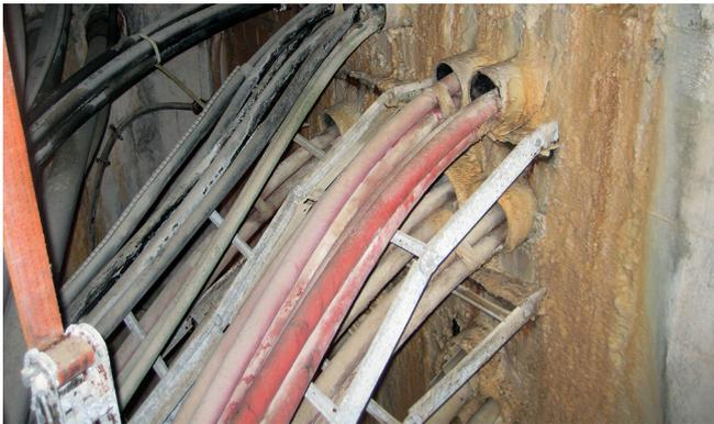
Siphon water intake before redevelopment: water ingress between wall sleeves and cables and between wall sleeves and wall.
