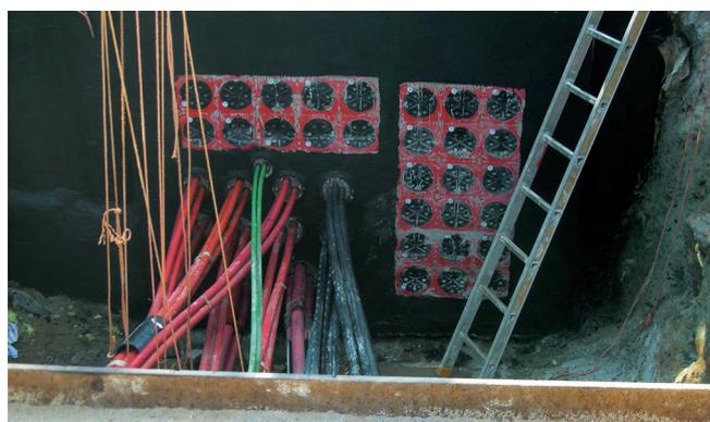
The wall of the siphon water intake was treated with a plastic modified thick coating.
