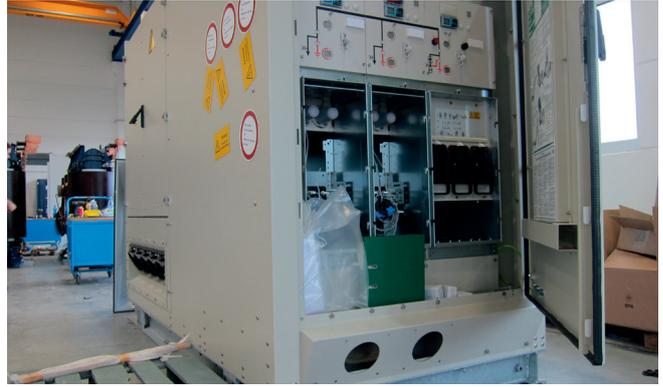
Final installation of the inverter station at the manufacturing facility.
