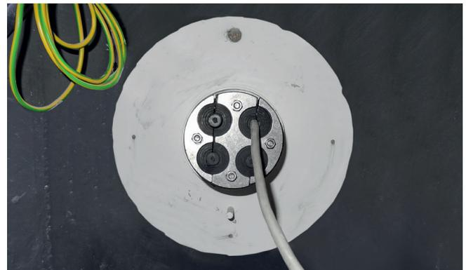
Installed cable in the partition S90 system HSS between the tribune and the technical room
