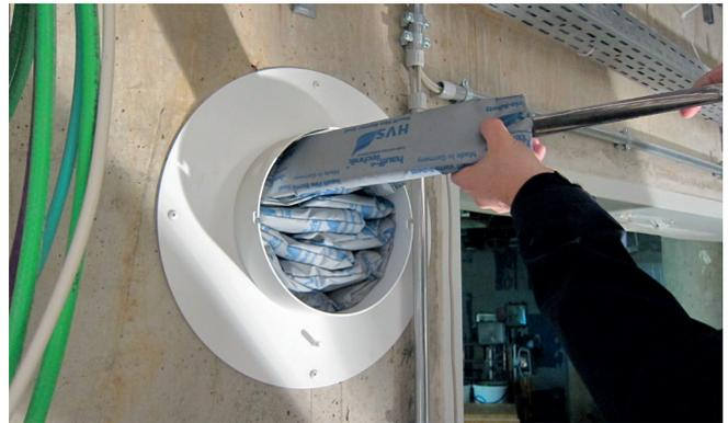
Installation of HVS fire-stop pads with the help of the assembly plate
