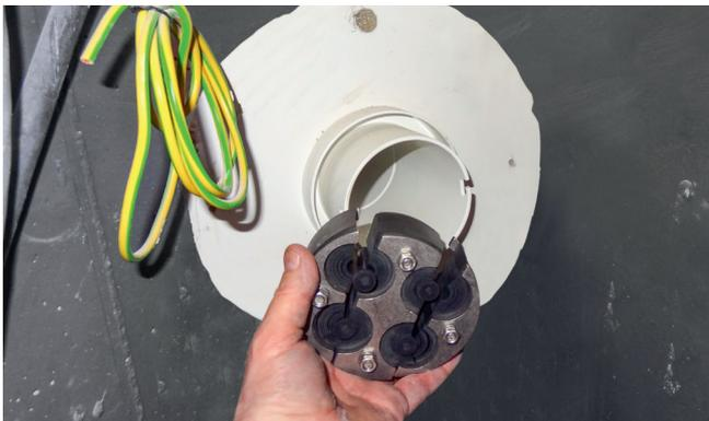
Installation of the partition HSS with a pressure tight cable sealing type HRD 100-SG in combination with the HSS fire-stop pads from one side
