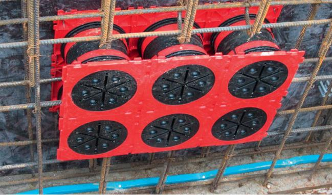
double wall insert HSI 150-K2 fixed as a package into the formwork
