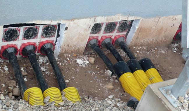
cable sealing with heat shrink method
