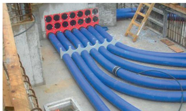
Cable entry system KES-M 150 with spacer for fixation and positioning of the hose bundles.
