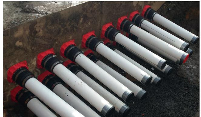
Connection of rigid Telstra conduits to HSI 150 wall inserts using KES-M 150-D system cover
