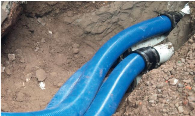
Connection of Hateflex spiral hose to rigid Telstra conduits
