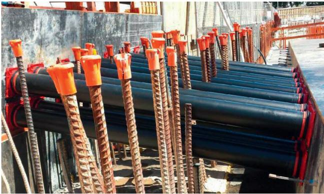
HSI 150-K2 wall insert 2,100 mm – mounted in formwork
