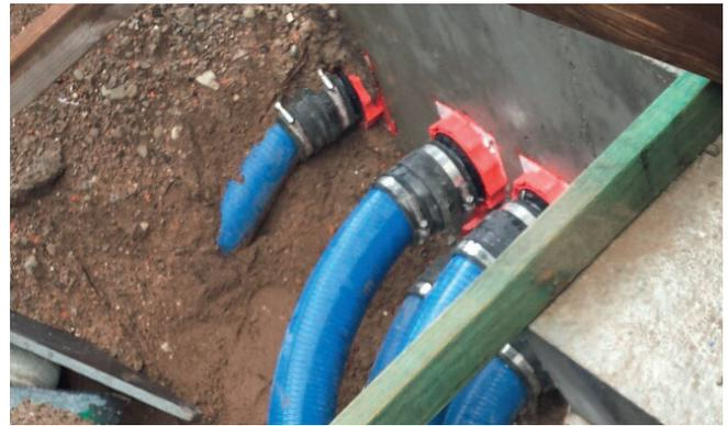
Connection of Hateflex spiral hose using KES-M 150-D system cover
