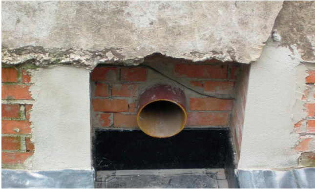
SML pipe sleeve - preparation of the stainless steel wall sleeve with fixed and loose flange type HRD-FUF.
