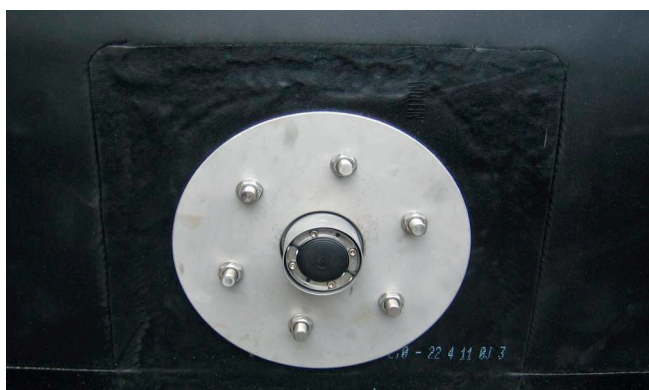
Wall sleeve HRD100-FUF after connection of the bitumen sheeting inclusive press seal HSD 100-SSG-18-65-SL V2A/EPDM.
