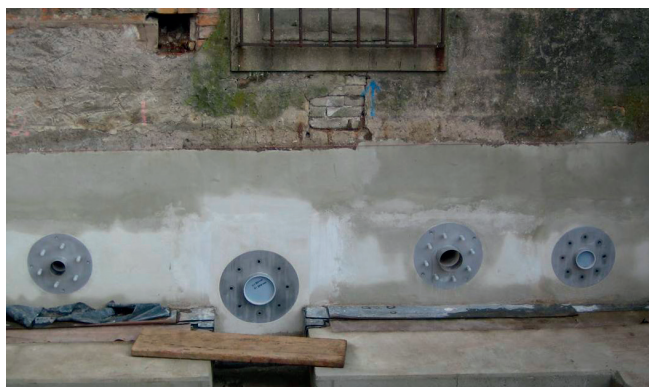
Wall sleeve HRD-FUF and HRD-FUFA diam. 100, 150 and 200 mm for entry of the supply lines.
