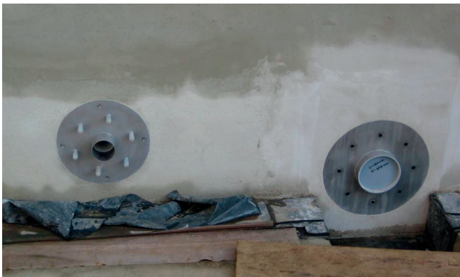
Stainless steel wall sleeve HRD-FUFA (for dowelling left side) with surface flush and cleaned clamping range.
