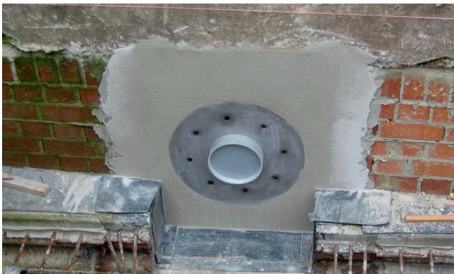
HRD-FUF was positioned eg concreting in with help of a connection sleeve.
