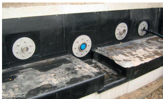
View on plinth wall and masoned basement wall after finished surface sealing, connected house entry according to DIN 18195 part 9 and before installing the new supply lines.
