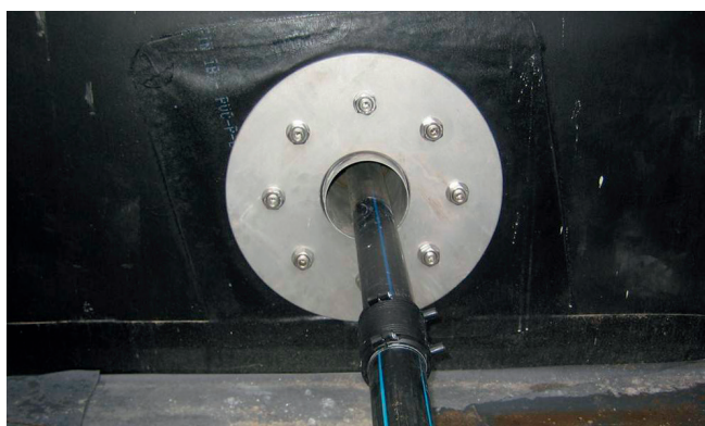
Wall sleeve HRD-FUF installed on the bituminous sheeting and inserted PE pipe DN32 with welded sleeve.
