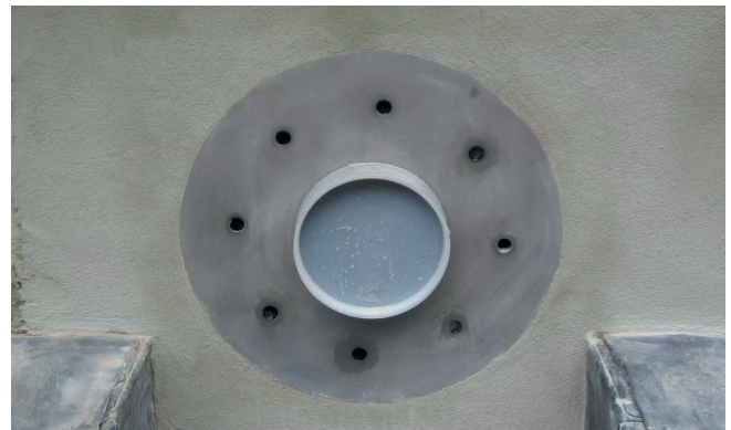
After concreting in the wall sleeve HRD 200-FUF. Preparation for flush connection of waterproof membrane.
