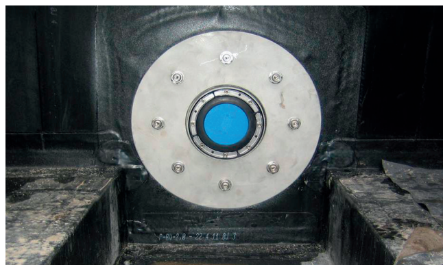
Wall sleeve HRD-FUF completely installed with press seal HSD 200-SSG-110-160-V2A/EPDM.
