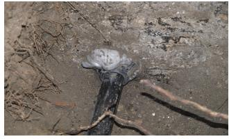
Inspection opening on outside of building: the completely escaped/partially exuded resin under the shield enables the integration of pre-existing surface sealing where applicable.
