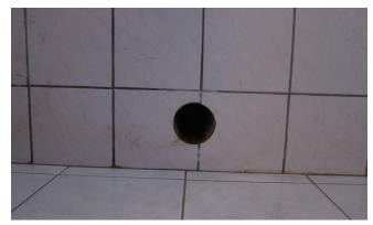
Refurbishment of building connections in existing buildings. Difficult conditions due to different basement constructions and construction materials. Making a core drill hole of 99-103 mm.
