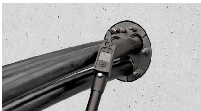
HRD150 PV G in kernboring
