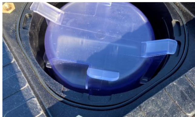
The integrated termination point in the box enables simple storage of the pigtails and connection of the cable systems in the G-Box. It also serves as a measurement point for the distance between the G-Box and PD.
