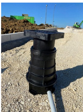
The height can be variably adapted thanks to the flexible G-Box. Simply pulling is sufficient to define the optimal installation height.
