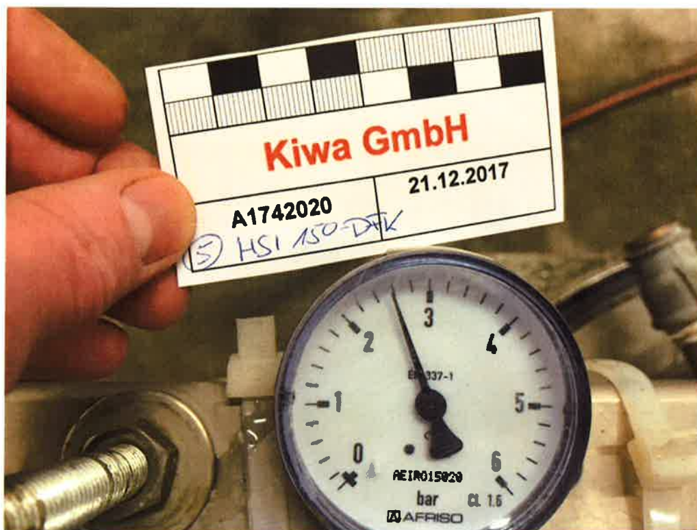
Figure A5. Water tightness test with \geq 2,5 bar water filled test cylinder (manometer at the beginning of testing on 21.12.2017).
