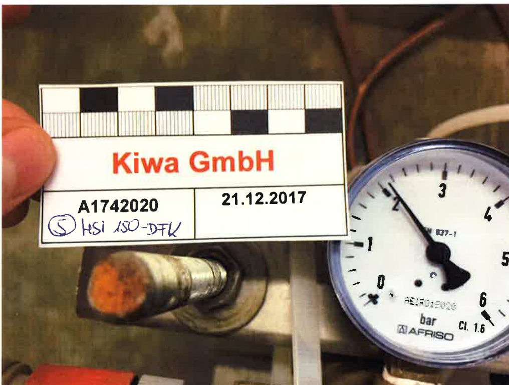
Figure A4. Water tightness test with \geq 2,0 bar water filled test cylinder (manometer > 24 hours on 21.12.2017).
